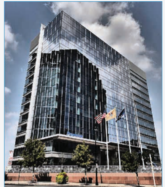
Panasonic's new North American headquarters at Two Riverfront Plaza was built with a commitment to environmental stewardship. By achieving energy costs 15 percent below the state's current energy code, Panasonic qualified for $440,459 in Pay for Performance incentives.
